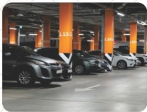
COVERED CAR PARKING
